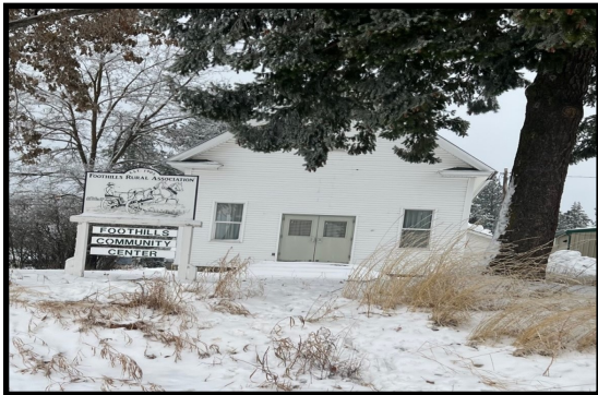
Street view of Center. Door can be used for emergency exits
